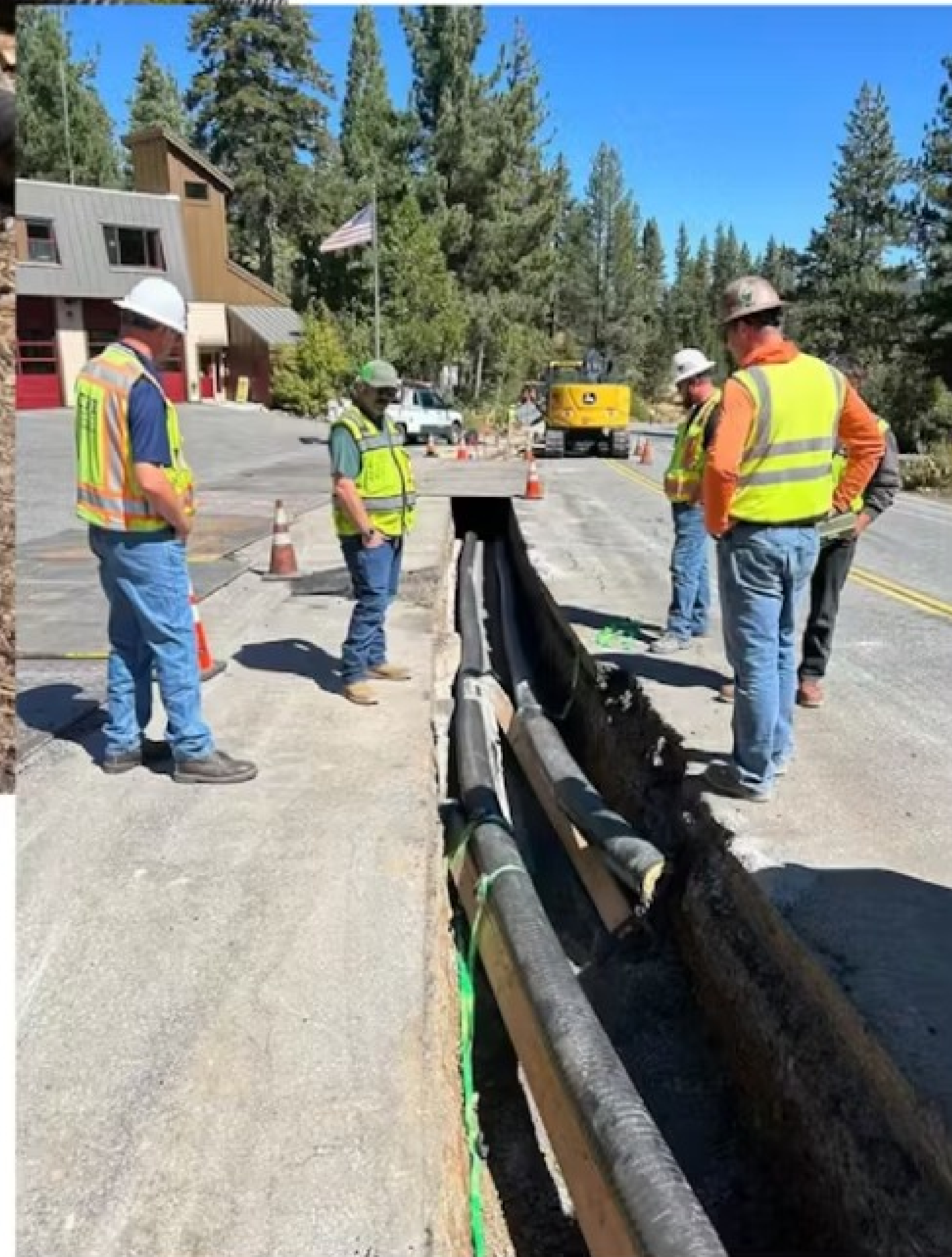
Insulated piping for heat distribution
