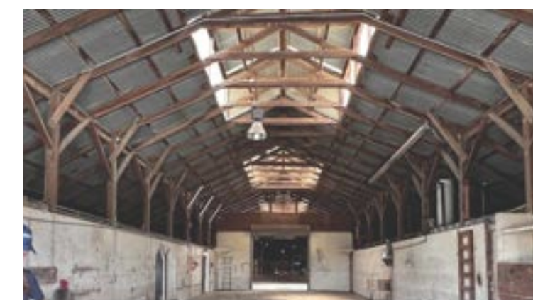
Figure 1.7: North extension of the barn
