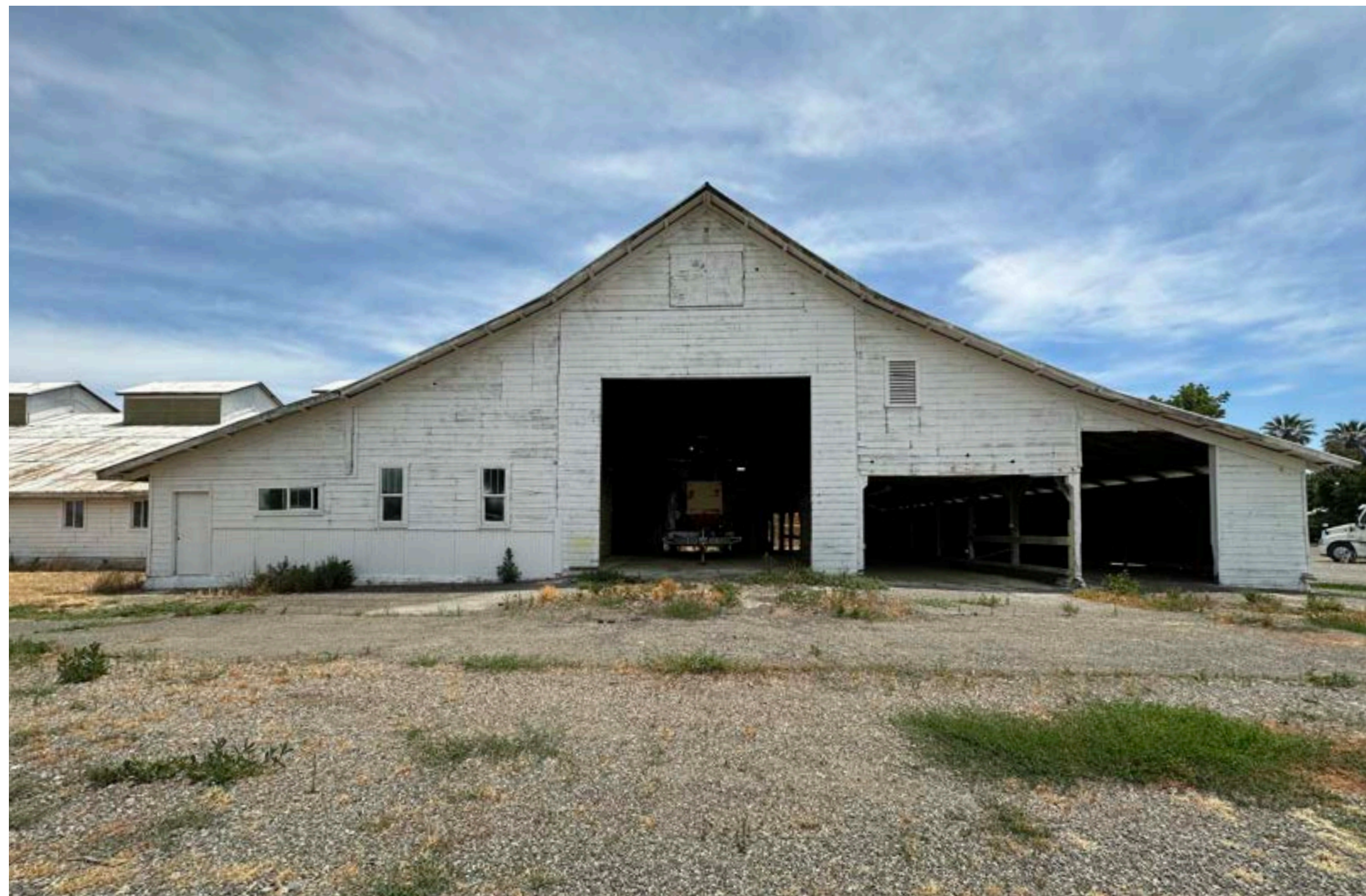
The barn's existing condition
